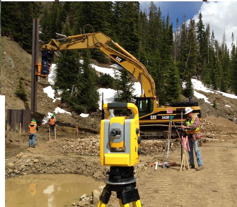
Above: Acklam's Will Spencer Jr. sets stakes for the centerline of tunnel alignment at the entrance portal.
