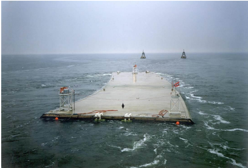
Figure: Off shore transport Tunnel elements on the North Sea
