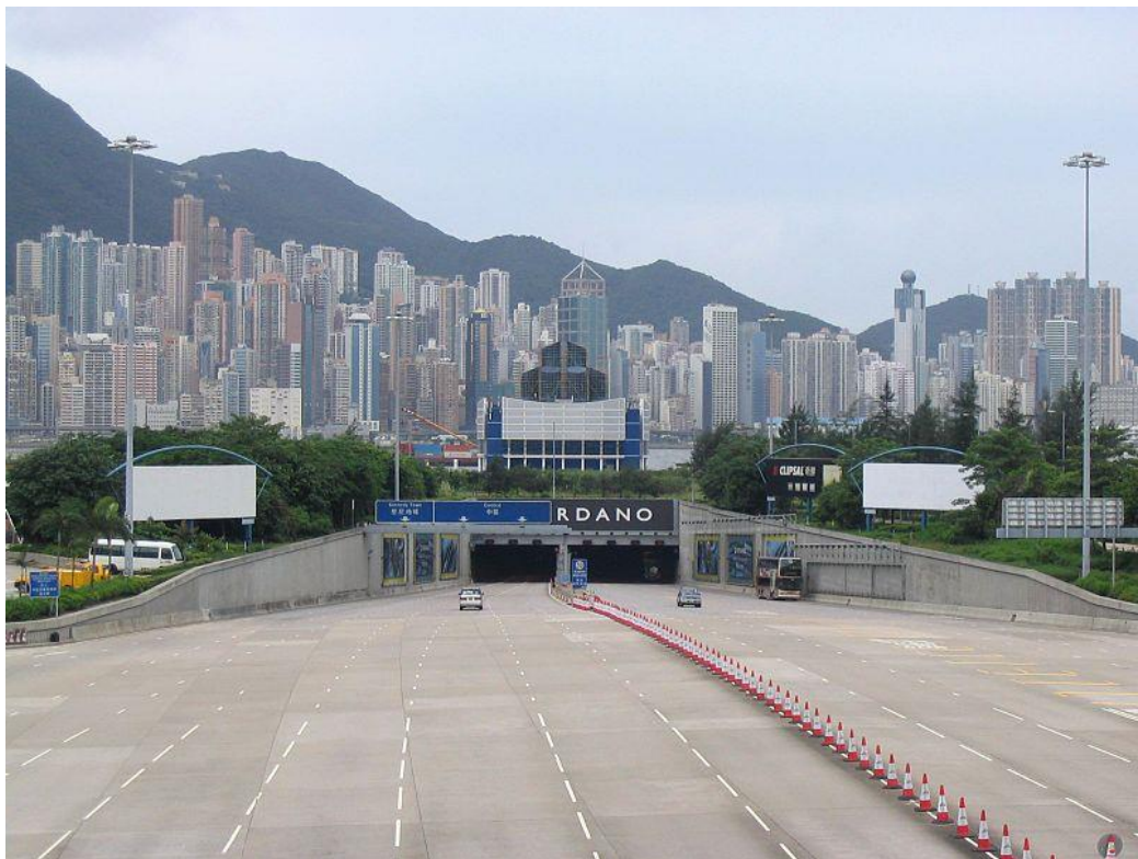
Figure: tunnel in operation (source: internet)
