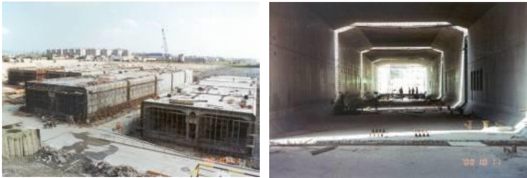
Figure: Tunnel elements under construction
