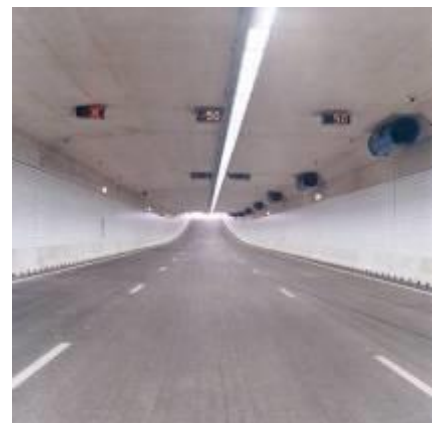
Figure: Tunnel interior
