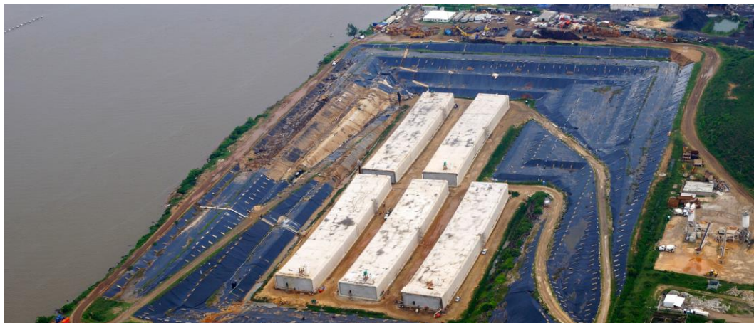
Figure: Tunnel elements under construction
