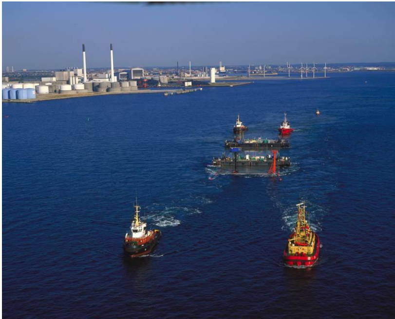
Figure: Transport of tunnel element
