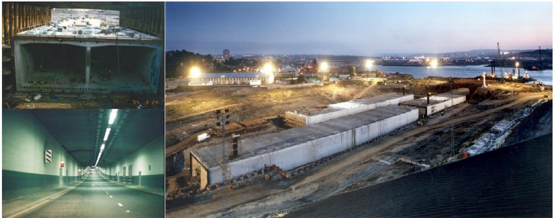
Figure: Medway tunnel under construction (top left, right) and completed (bottom left)
