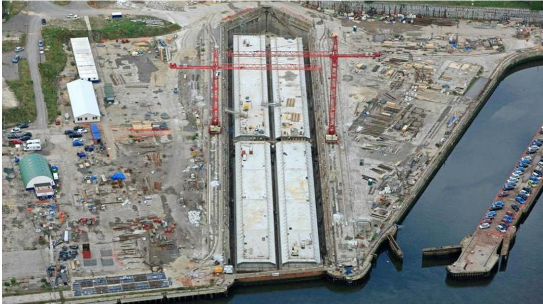
Figure: Tunnel elements in the construction dock (ship yard in Newcastle)
