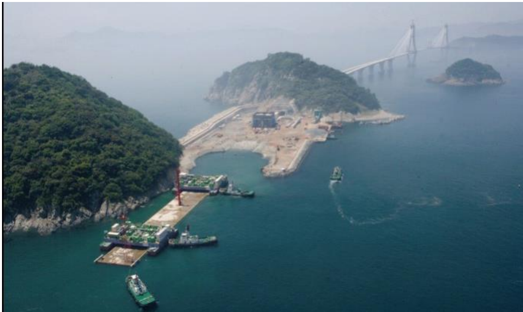
Figure: Bridge – Tunnel transition
