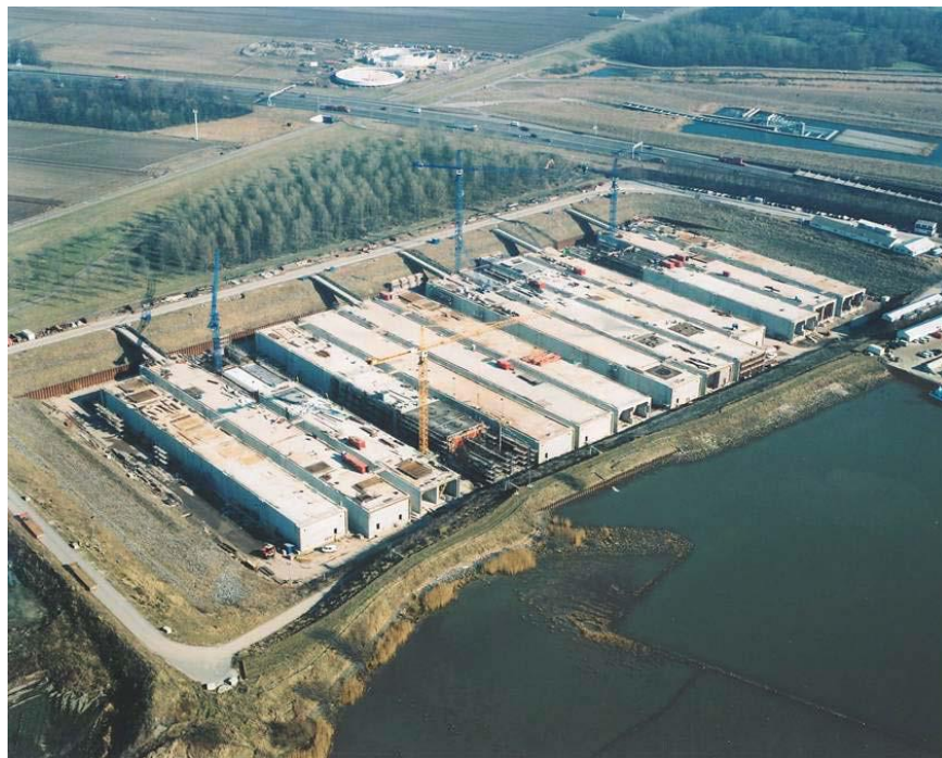
Figure: tunnel elements for crossing with river Oude Maas and Dordtsche Kil in construction dock
