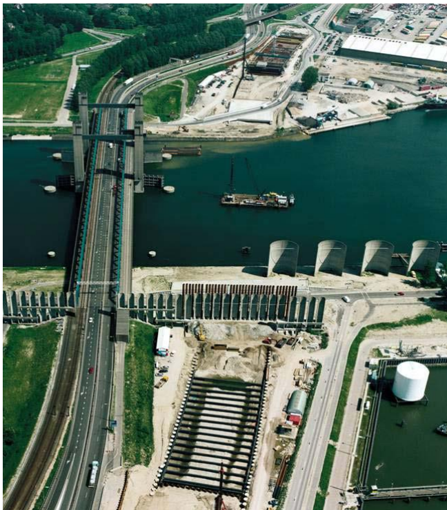
Figure: Tunnel under construction
