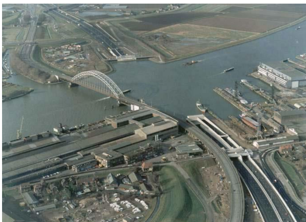
Figure: Tunnel under the river Noord
