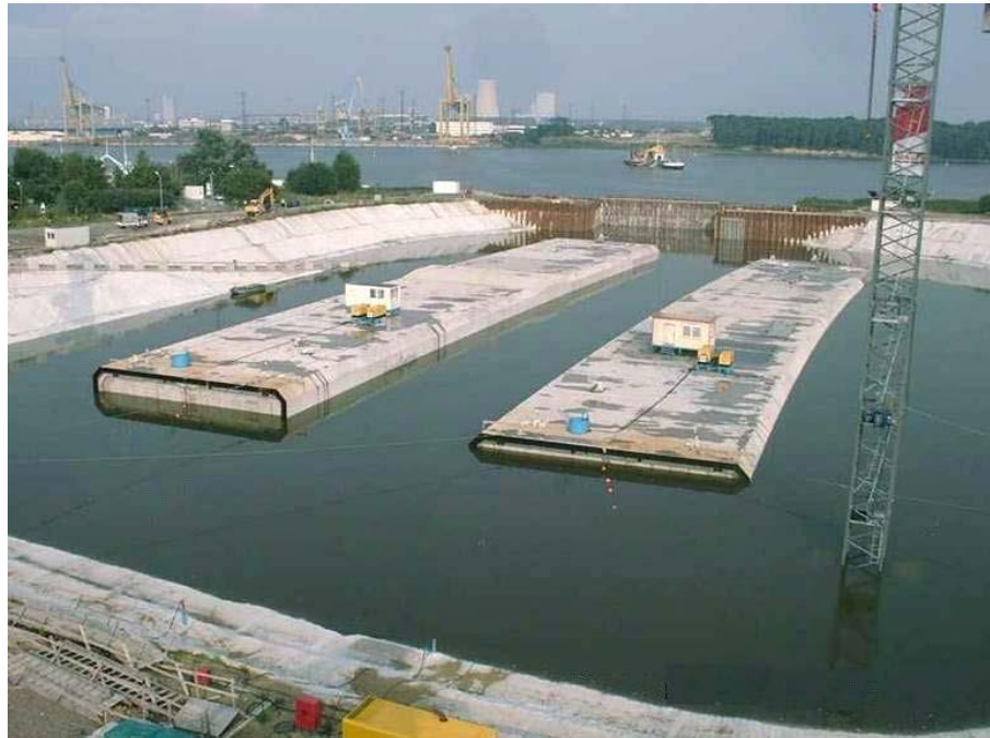
Figure: Tunnel elements floating in construction dock
