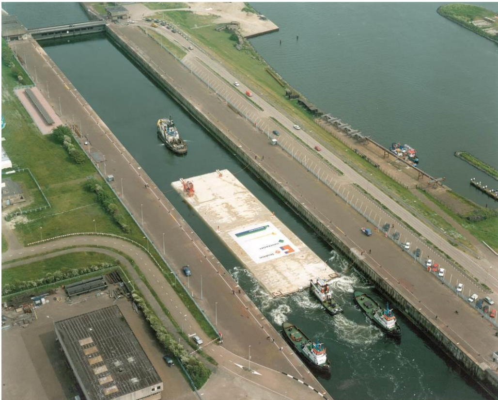
Figure: transport tunnel elements
