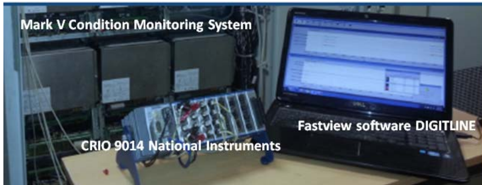
Fig.2. The experimental setup for control room measurement data
