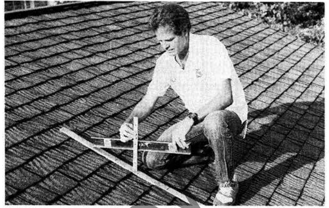
Figure 1-15 Determining roof slope
