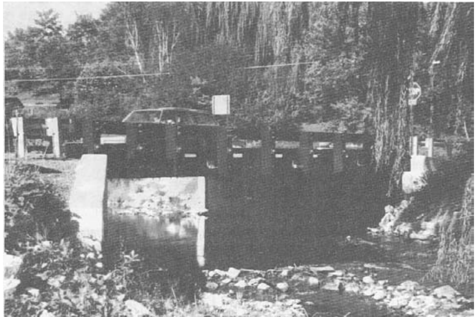
Figure 2-28- Stress-laminated deck bridge built near State College, Pennsylvania, in 1987. The bridge is 28 feet wide and was constructed from 4-inch-wide by 16-inch-deep lumber laminations.
