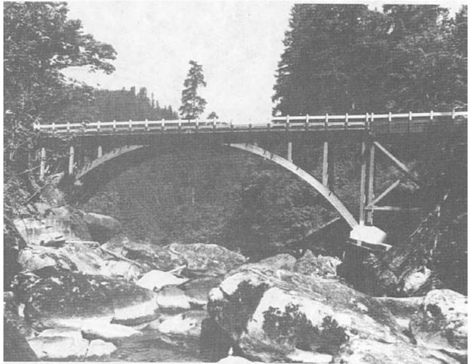
Figure 2-19.-- The Loon Lake Bridge is a three-hinge glulam deck arch design, built near Roseburg, Oregon, in 1948. The bridge spans 104 feet and supports a 20-foot roadway.
