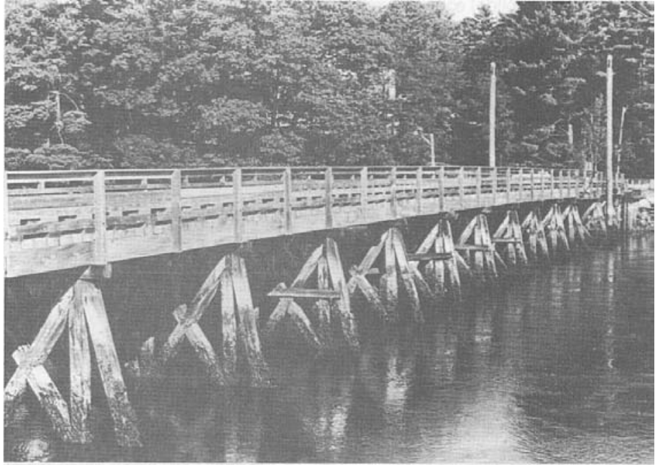
Figure 2-16.- Sewall's bridge is a timber trestle vehicle bridge in York, Maine. The bridge was built in 1933 using the same design features of the original bridge, built in 1761, that it replaced. This bridge became a designated landmark of the American Society of Civil Engineers in 1986 (photo courtesy of the American Society of Civil Engineers; Used by permission).
