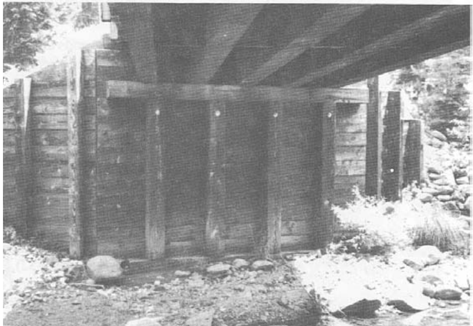
Figure 2-31.- Sawn lumber post abutment.
