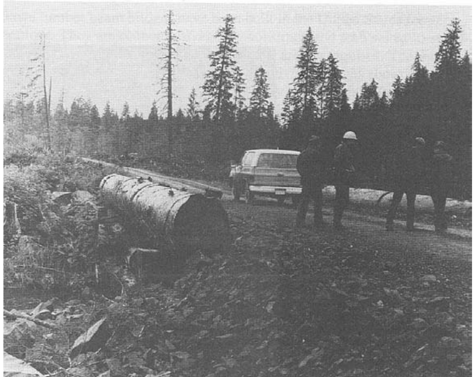
Figure 2-3.- Log beam bridge with a gravel deck. The two large “brow” logs along each side serve to delineate the roadway and function as a type of railing.
