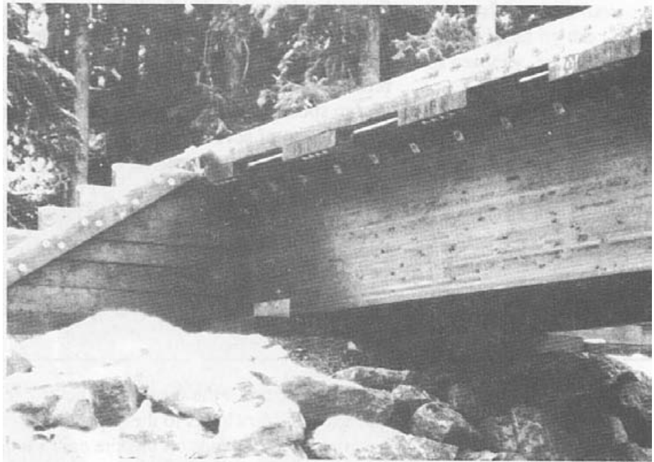
Figure 2-30.- Surface bearing spread footing constructed of glulam (photo courtesy of Tim Chittenden, USDA Forest Service).
