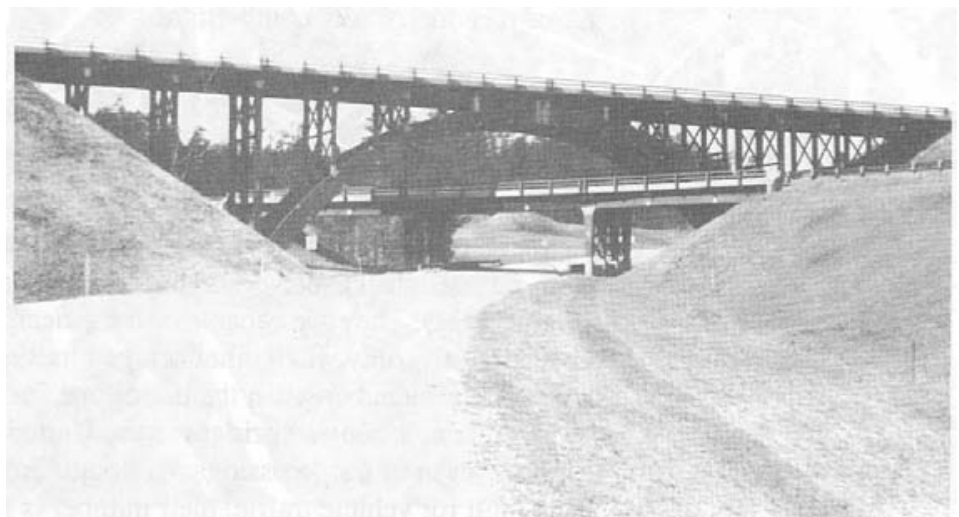
Figure 2-20.- Three-hinge glulam deck arch bridge at the Keystone Wye interchange off U.S. Highway 16, near Mount Rushmore, South Dakota. The arch spans 155 feet and supports a 26-foot-wide roadway (photo courtesy of Wheeler Consolidated, Inc.).
