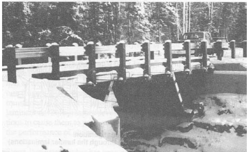
Figure 2-29.- Stress-laminated deck bridge with stress-laminated slant-leg supports, built near Espanola, Ontario, Canada, in 1981. The bridge spans approximately 55 feet and supports two traffic lanes (photo courtesy of the Ontario Ministry of Transportation).
