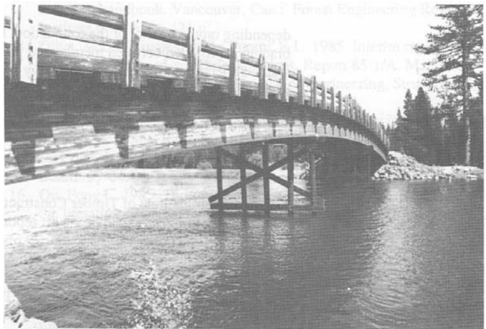
Figure 2-33.- Timber pile bents.
