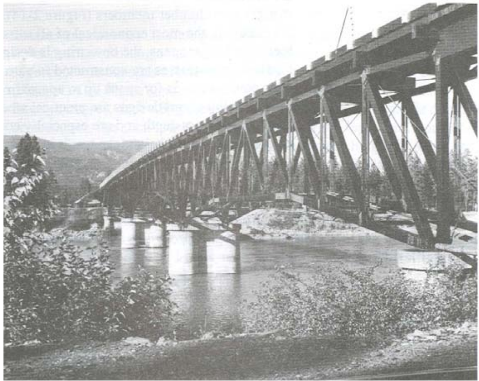
Figure 2-15.- A multiple-span parallel-chord deck truss bridge.
