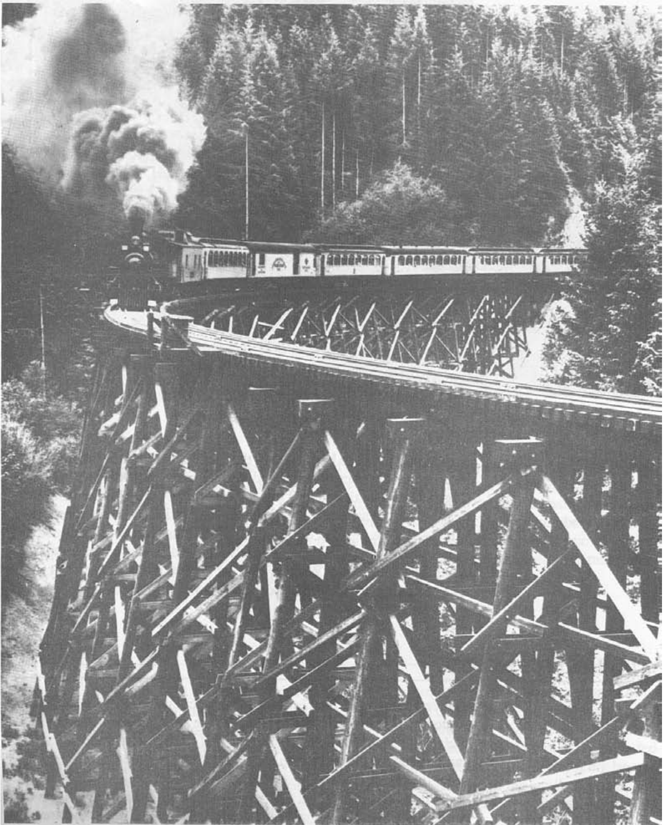
Figure 2-17.- Early railroad trestle on the Verona, South Park, and Sunset Steam Railroad. Many long-span timber trestles of this type were built for railroad use, requiring large volumes of wood for the complex bent substructures (photo from the Forest Service Collection, National Agriculture Library).
