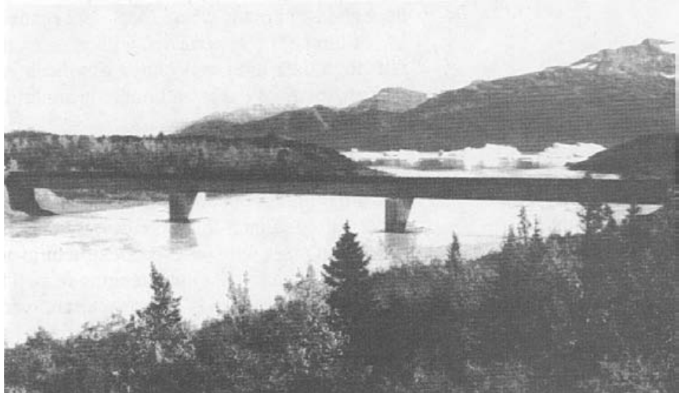
Figure 2-7.- Glulam beam bridge over Dangerous River, near Yukatat, Alaska. This bridge consists of three 143-foot spans, each of which is supported by four glulam beams that are 91-1/2 inches deep (photo courtesy of the Alaska Department of Transportation and Public Facilities).
