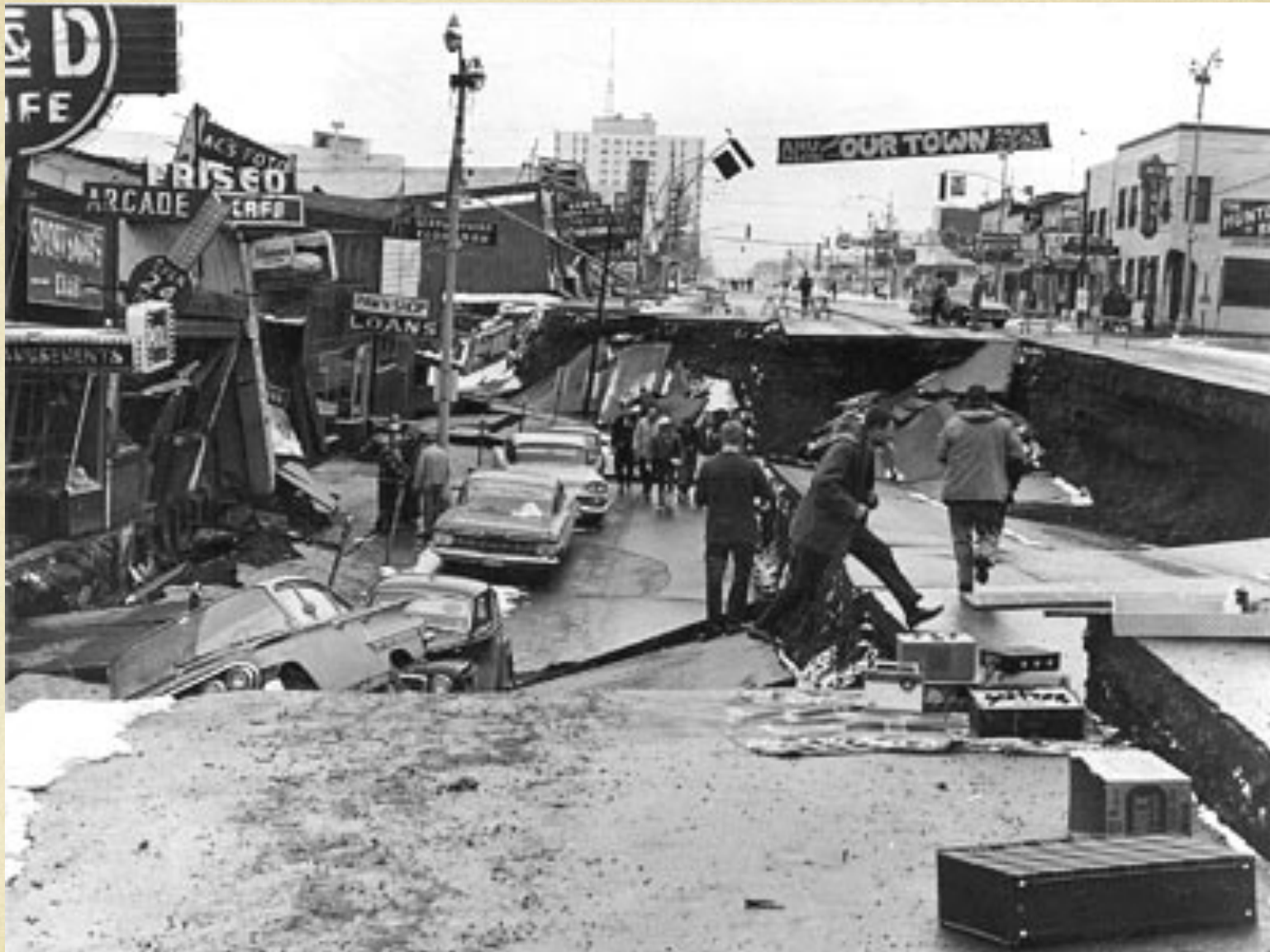
Earthquake damage in Anchorage on March 27, 1964
