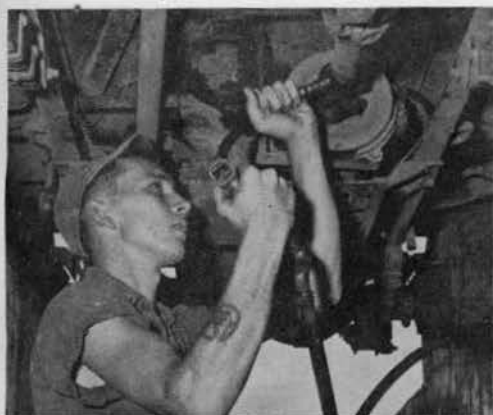
GREASE RACK - Using the grease gun to oil the drive shaft on an "A" Company vehicle on the grease rack at the compound area is R.B. Cox, CM3.
