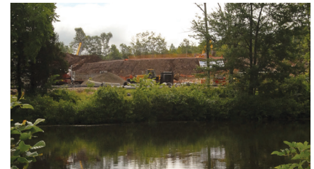
The new Armed Forces Reserve Center serves as a “virtual installation” for Army Reserve soldiers from Maine to Virginia (top). Construction of the new building prompted wetlands mitigation efforts (bottom).
