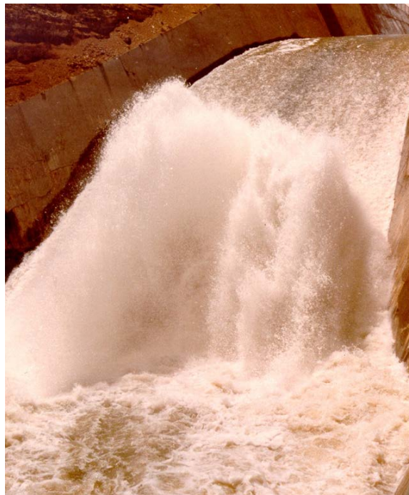
Figure 9. Rooster tail during spillway releases
