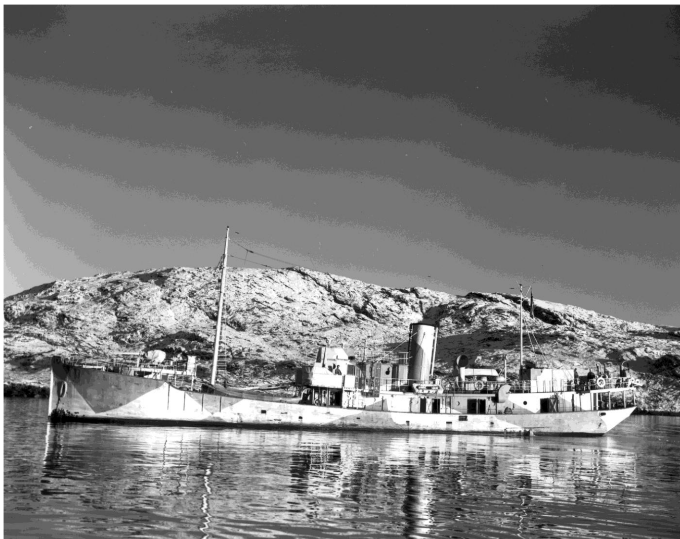
WYP-172 Alatok 19Mar1943 -- probably off Greenland
