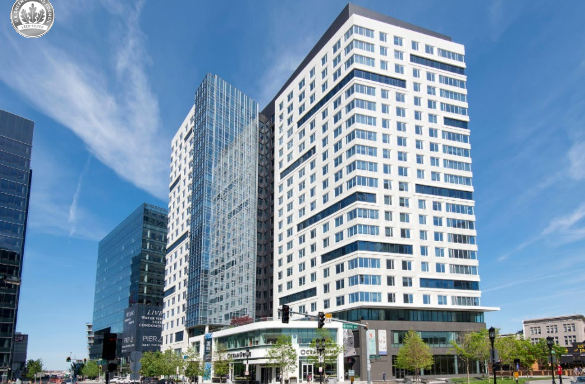
100 Pier 4 | Boston, MA
