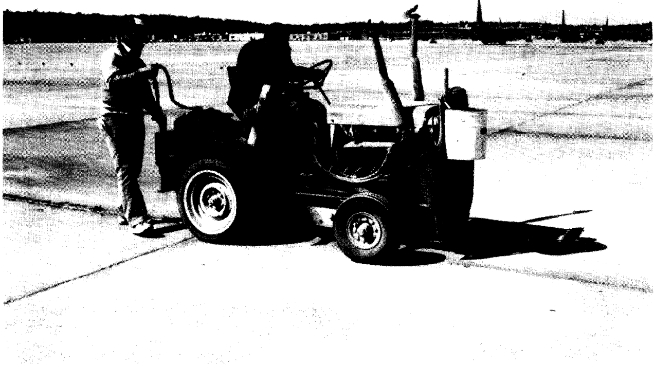
Figure 4-3. Joint Plow Removing Old Sealant.
