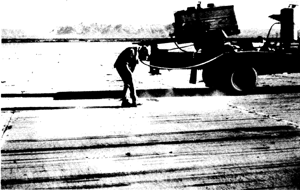
Figure 4-4. Sandblasting Equipment Cleaning Joints.
