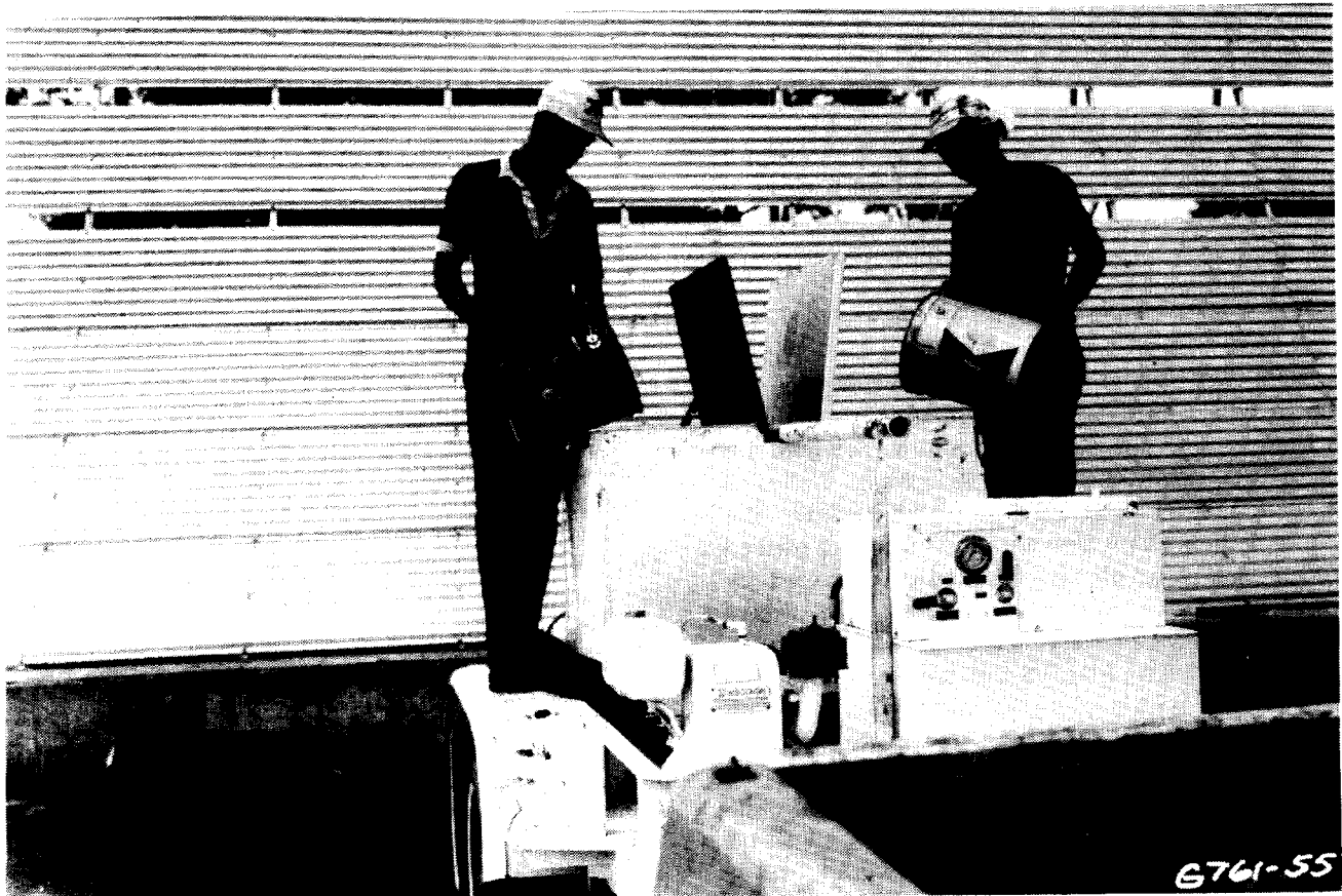
Figure 5-3. Cold-Applied, Two-Component Sealant Application Equipment.
