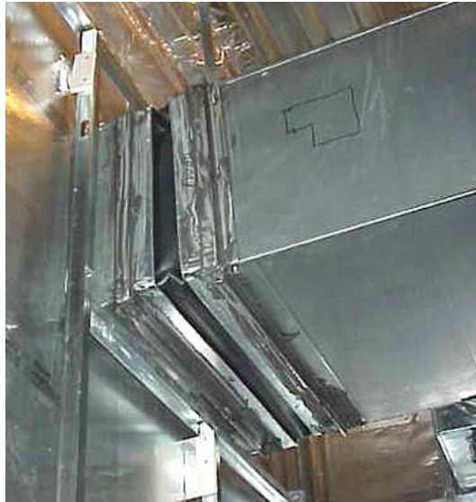
Figure 3-6 Duct Penetrations
