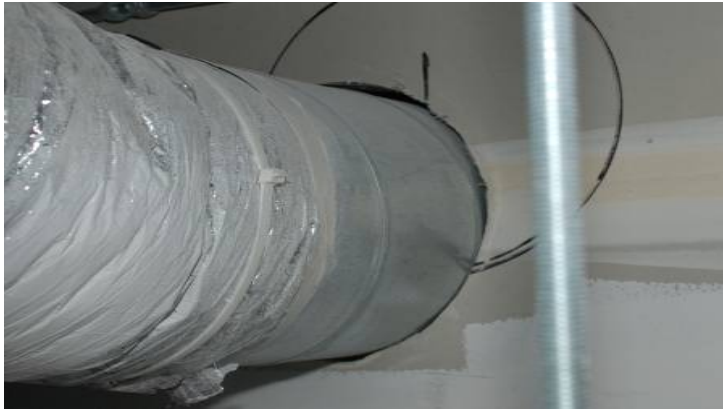
Figure 3-7 Sealing Penetrations
