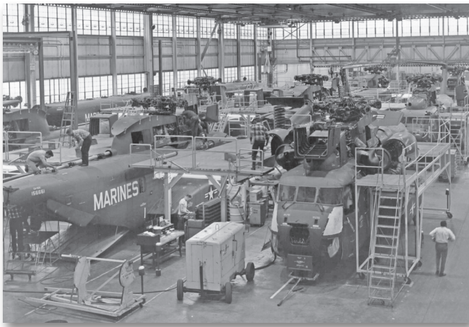
CH-53D production at Stratford delivered 124 improved Sea Stallions to the Marines, plus export aircraft for Israel and Austria. Similar CH-53Gs were co-produced in Germany. (Sikorsky Archives)
