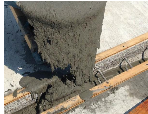
Deck-level connection between precast deck panels.
