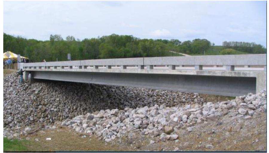
Mars Hill Bridge, Wapello County, Iowa
