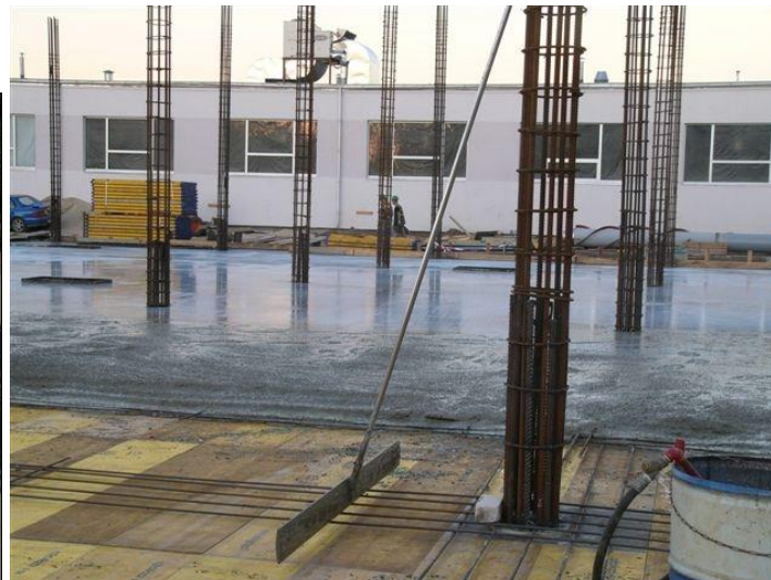
First floor, elevated slab
