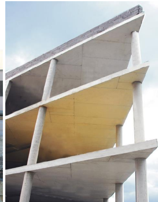
Elevated slabs (recent development)
