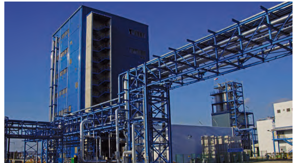
BASF plant in Yeosu, Korea
