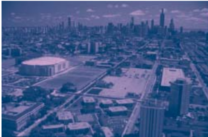
HOLMES HAS HAD A HAND IN THE SUCCESS OF MULTIPLE PUBLIC WORKS AND COMMUNITY PROJECTS IN CHICAGO. THE CITY'S HOWARD/DAN RYAN EL CONNECTOR PROJECT (ABOVE) IS JUST ONE EXAMPLE.
