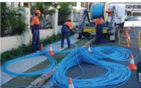
Figure 7 Cable stored in 'fig-8' shape
