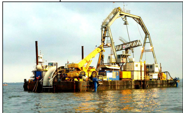
Figure 8: Submarine cable laying barge
