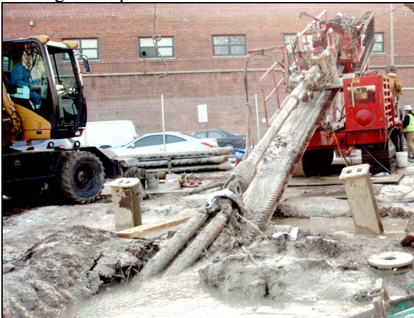
Figure 7: Horizontal directional drilling for conduit bundle
