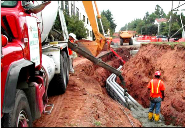
Figure 6: Open-cut trenching for duct bank installation
