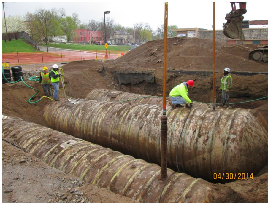
Above: A Des Moines May 2014 tank removal of three 12000 gallon fiberglass tanks.
