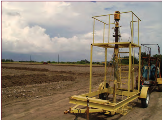
Figure 13. A dual grade laser gives the grade to the trencher.
