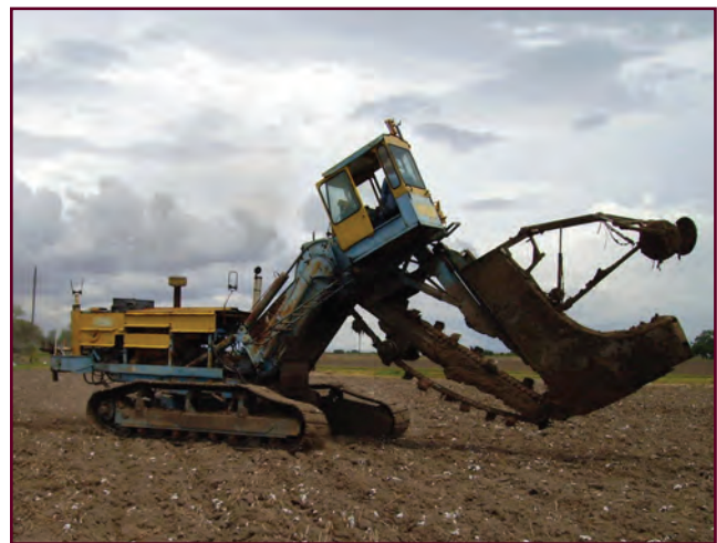
Figure 7. Moving the trencher to install the subsurface drain pipe.
