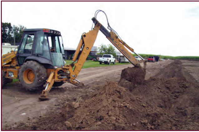
Figure 8. Digging a hole to start installing the subsurface drain.
