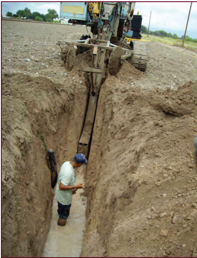
Figure 9. Installing an interceptor drain tile.
