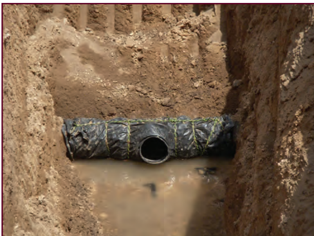
Figure 14. Collector drain tee.
