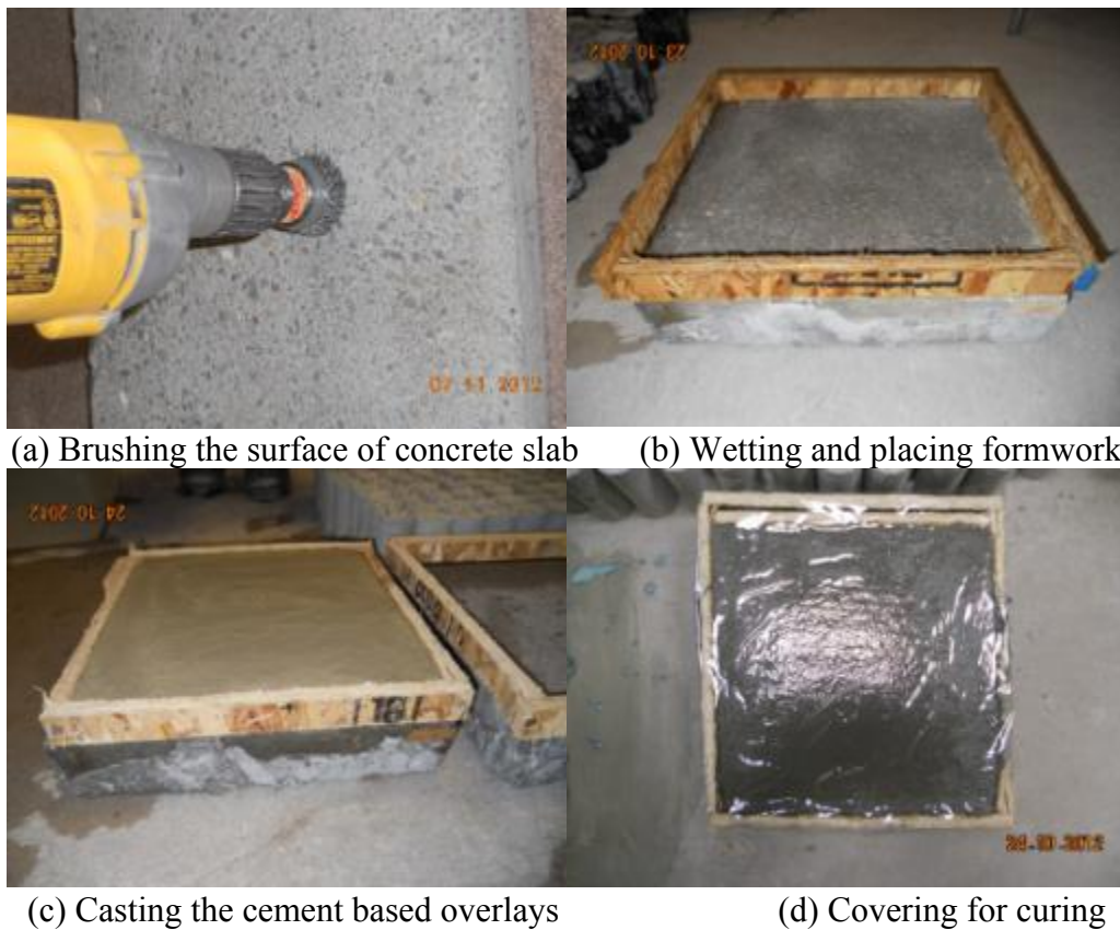
Figure 7.1: Preparation of the cement based overlays
