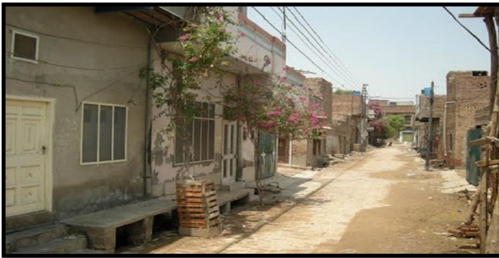
Photo 7.3: Variety of property sizes and building materials
