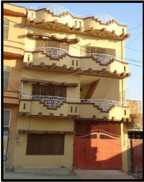
Photo 7.4: Modern facades and metal entrance gates
