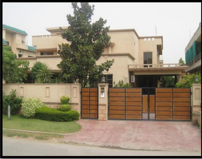
Photo 4.23: More than 25,000 sq.m. Properties, with servant quarters at the back
