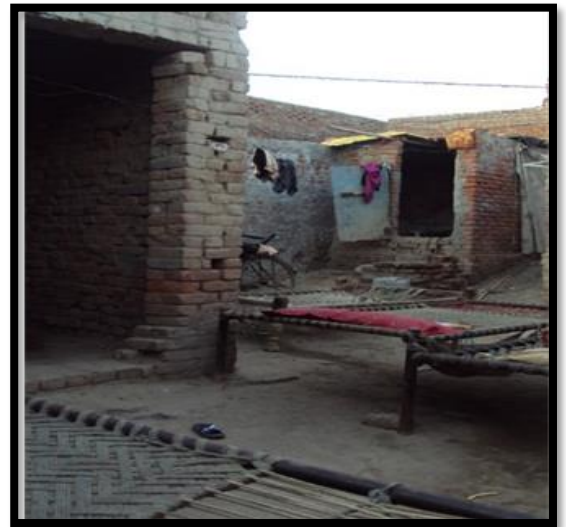
Photo 4.9: Haphazard additions to property
