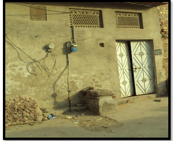
Photo 4.13: A relatively finished boundary wall
