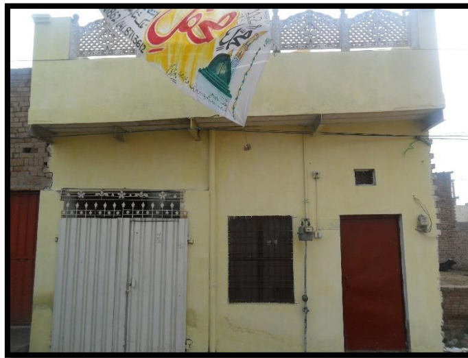
Photo 7.1: A completely rebuilt property
