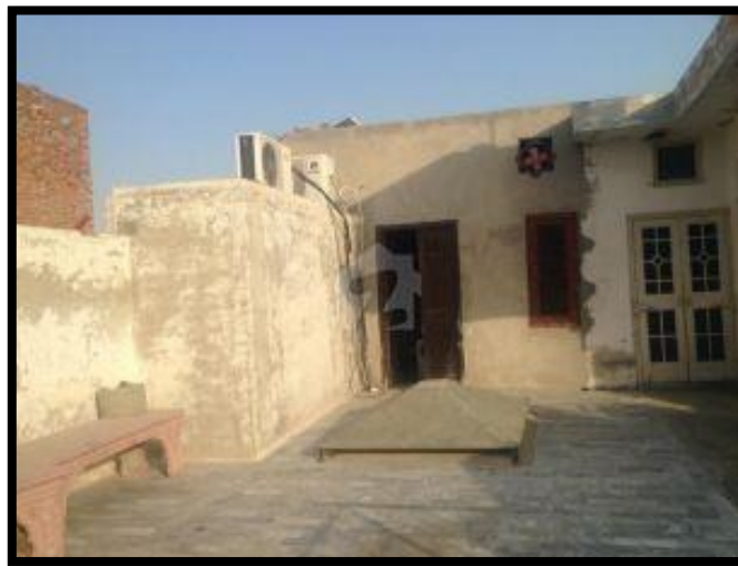
Photo 7.2: Incremental consolidation, addition of a room on the roof Source: Ali Real Estate Agents
