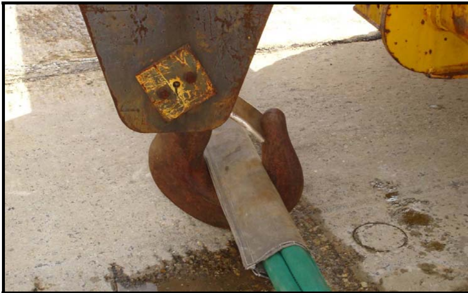
Figure 13. Using Protective Sheath to Protect Slings
