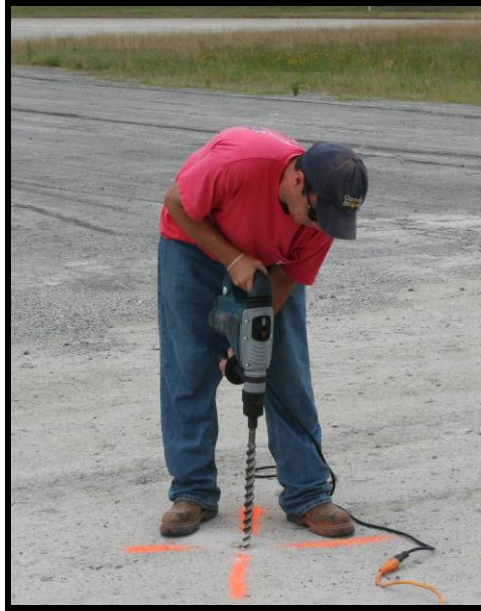
Figure 2. Drilling Through Overlying Stabilized Surface
