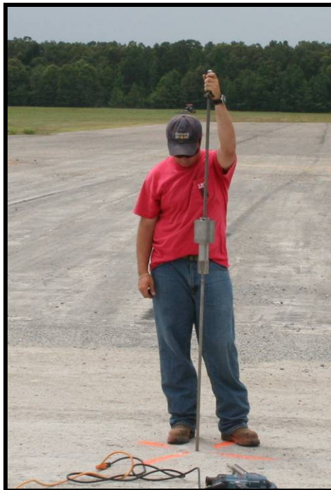
Figure 3. Using a DCP to Determine Subgrade Soil Strength
