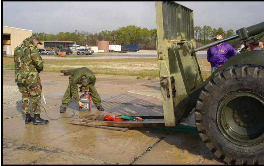
Figure 9. Drilling Holes for Anchor Bolts
