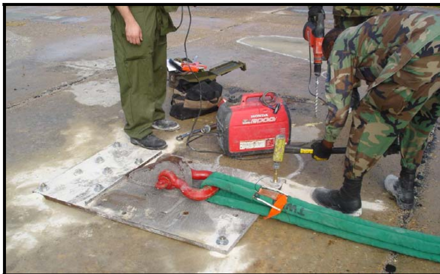
Figure 11. Complete Installation of Bolts
