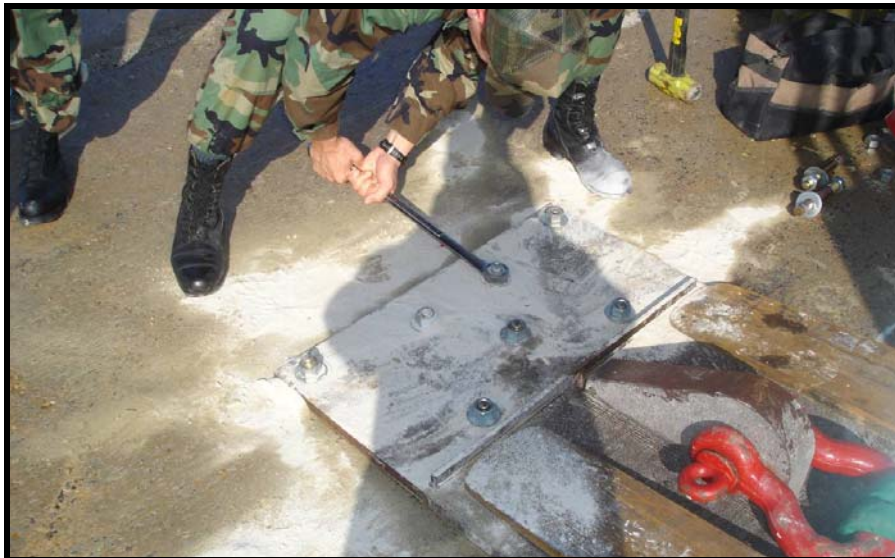
Figure 10. Securing Nuts on Anchor Plate
