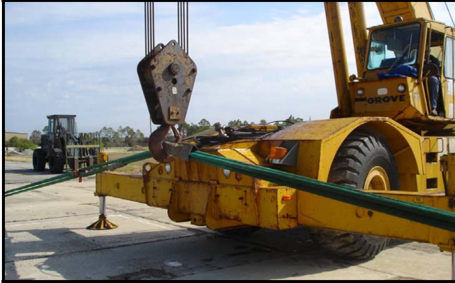
Figure 14. View of Crane Applying Load to Slings
