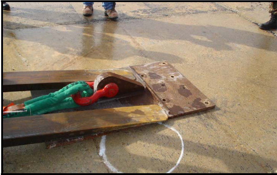
Figure 7. Positioning Anchor Plate with Forklift.
