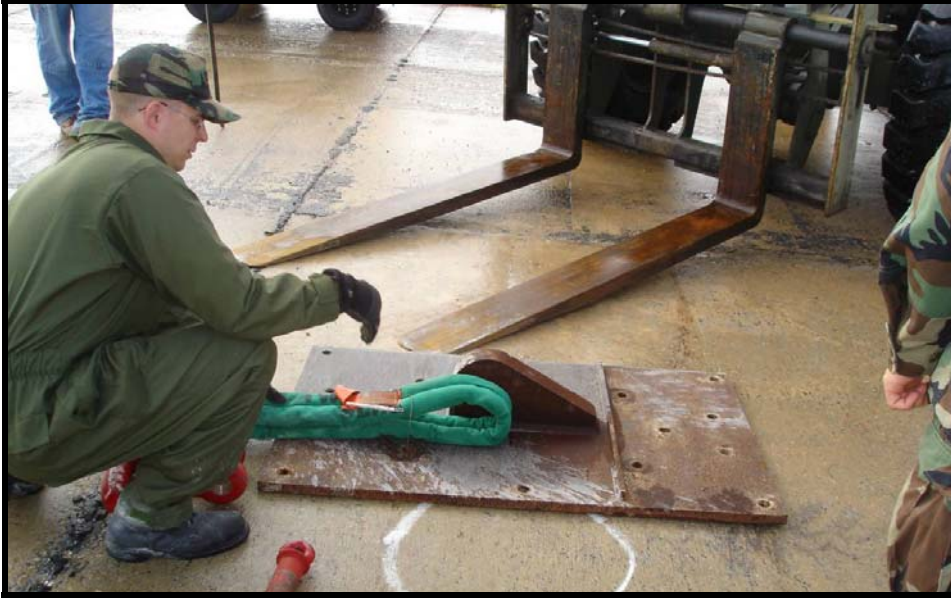
Figure 5. Position Anchor Plate and Connect Sling
