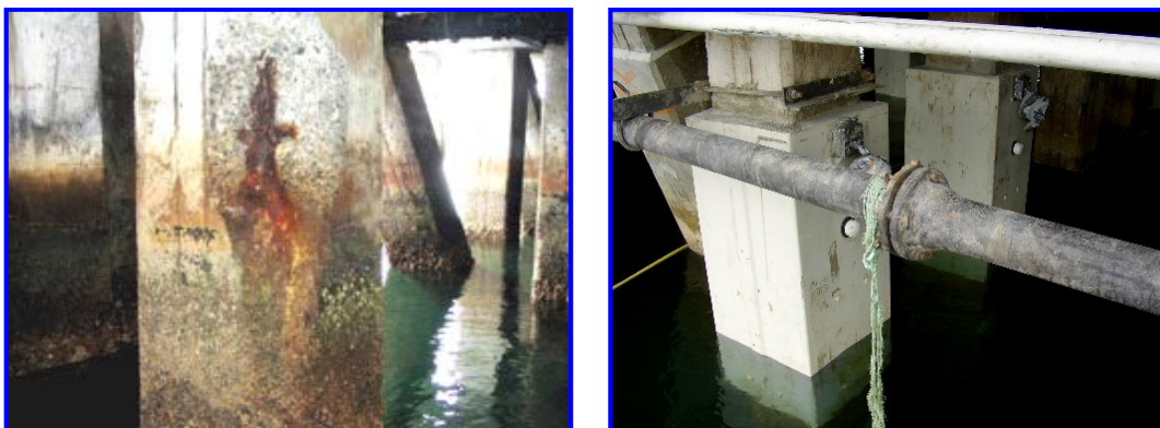
Figure B-29 Photos Showing “Before” and “After” Installation of Integrated Pile Repair and CP Systems
