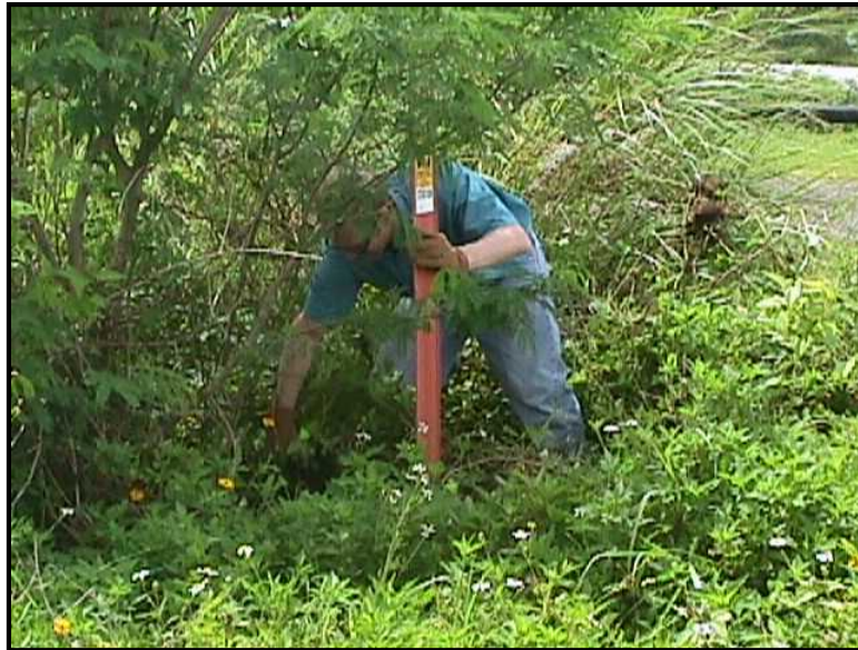
Figure B-13 Test Station Marker for Flush Mount Test Station.
