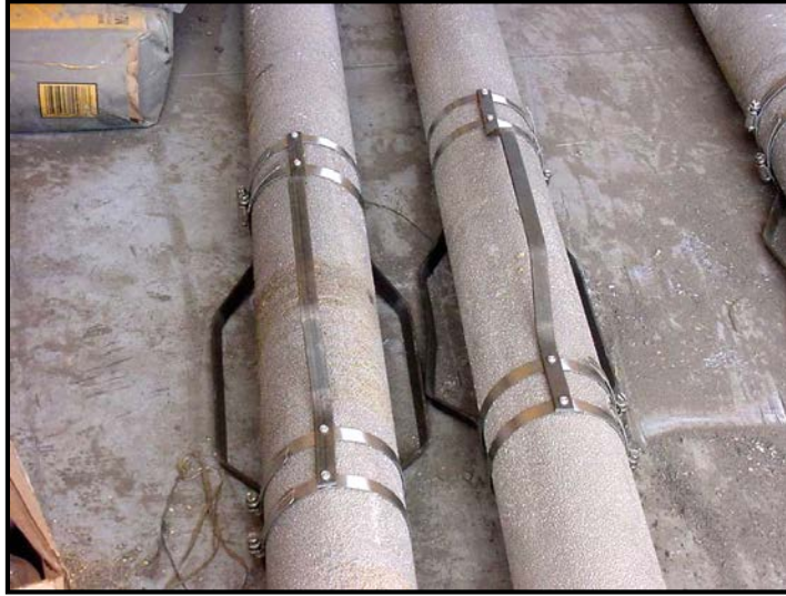
Figure B-22 Centralizers Installed on High Silicon Cast Iron Anodes
