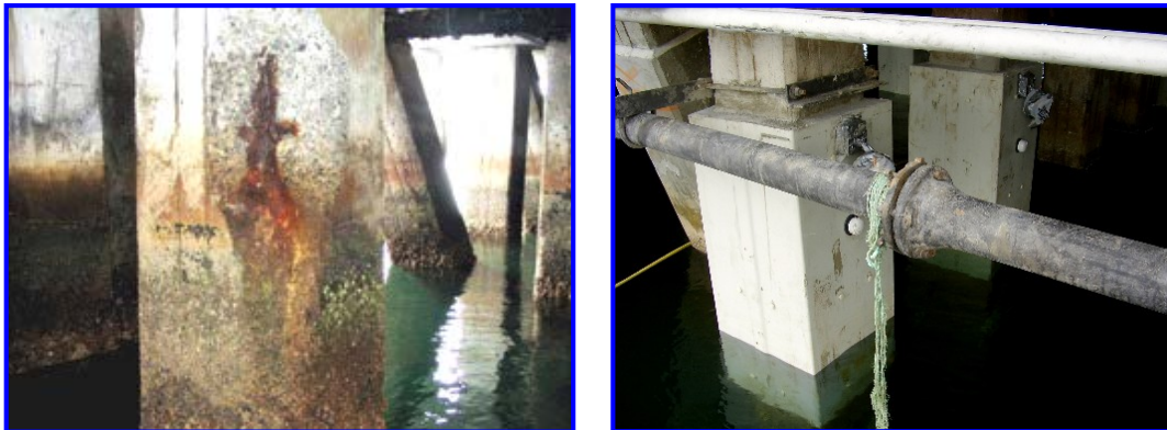
Figure 4-10 Photos Showing “Before” and “After” Installation of Integrated Pile Repair Systems
