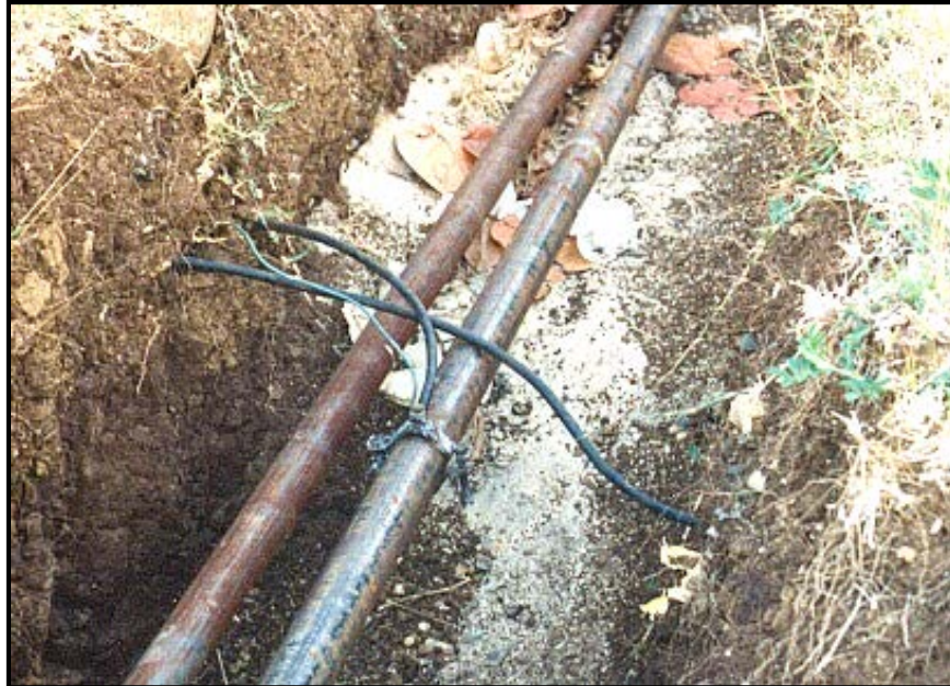
Figure 4-5 Mechanical Connection of Wiring to the Structure
