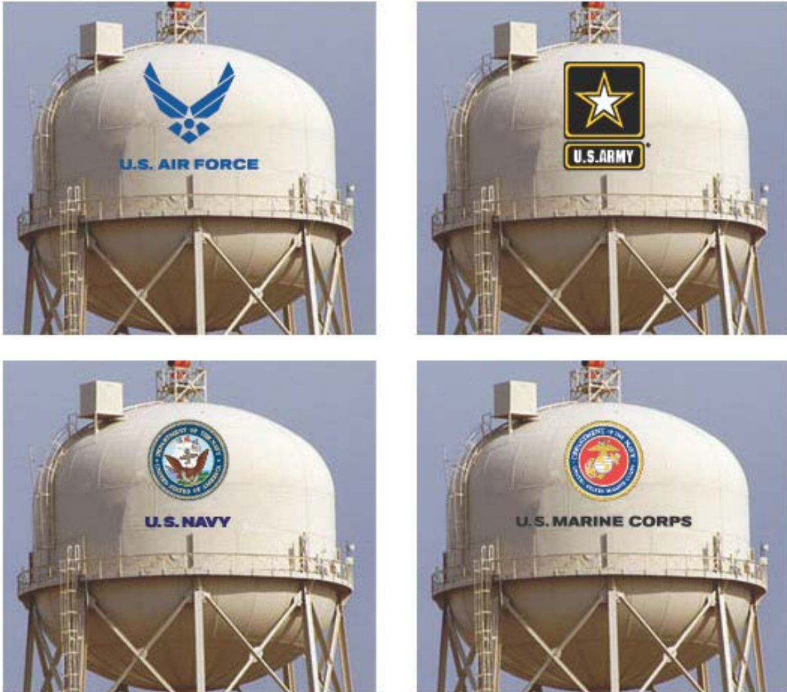
Figure 3-17 Water Tower Signs.
