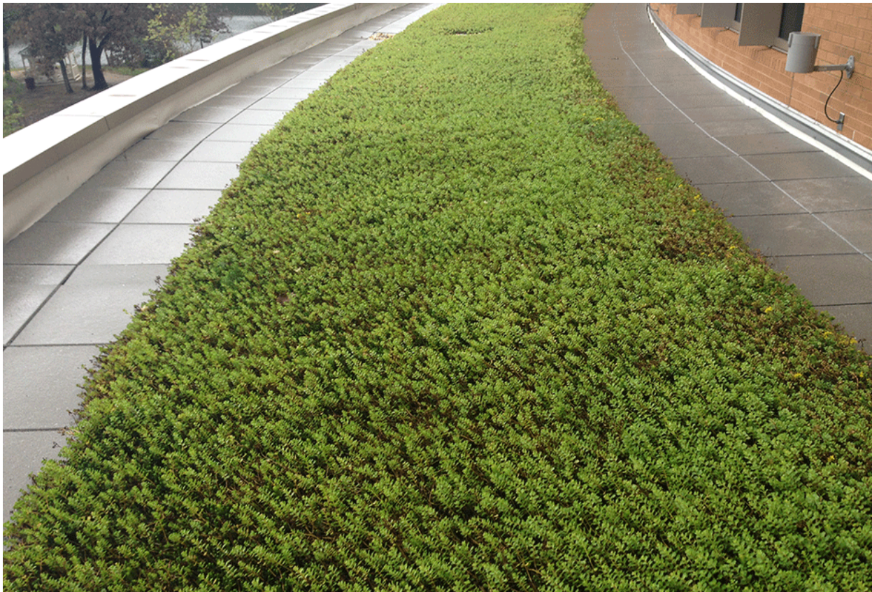
Figure A-3 Extensive Green Roof
