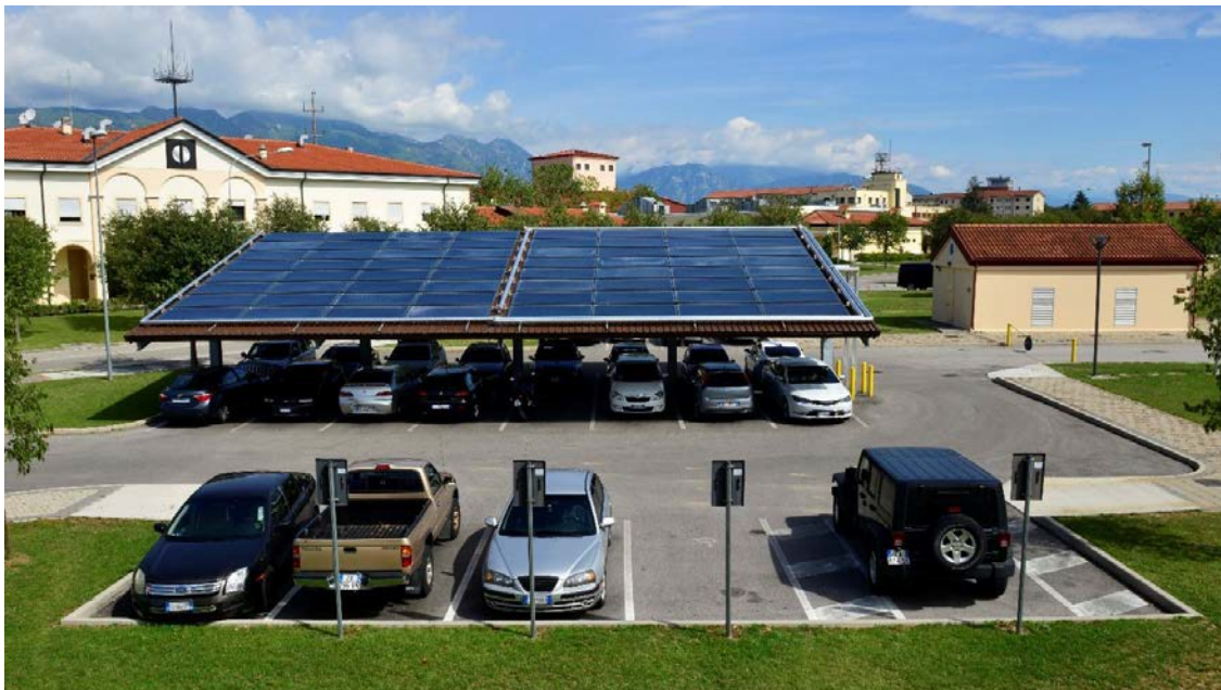
Figure A-5 Covered Parking: Parking Canopy with Photovoltaic Solar Panels 2
