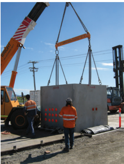
R8 hanger bar with hooks for 1.3t RA anchors
