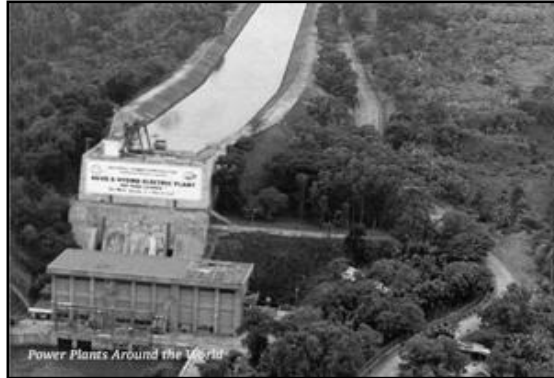
Photograph courtesy of National Power Corporation, retrieved from http://www.industcards.com/hydro-philippines.htm
