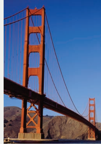
▲ Golden Gate Bridge
