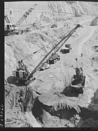
Steam Shovel and Dump
