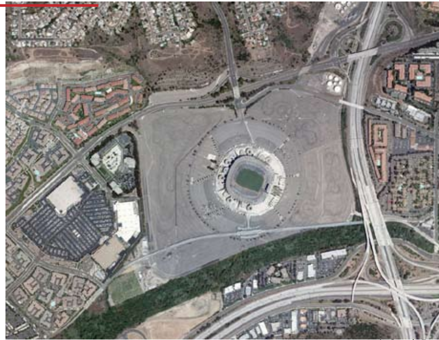
San Diego; Qualcomm Stadium Aerial (2, Google Earth)
