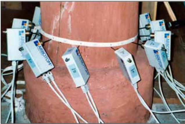
Figure 4.1—Acoustic tomography test on a timber post. (Rinn 2006)
