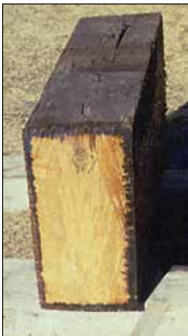
Figure 1.13 —Only the outer portion of this timber contains preservatives.
