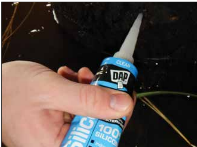
Figure 2.14—Silicone is used to fill the small drilling hole.
