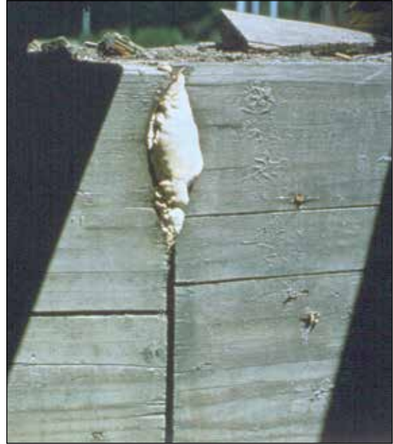
Figure 1.1—Fruiting body between two beams.
