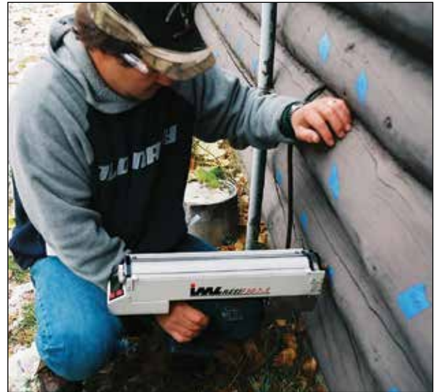
Figure 2.9—A resistance microdrill used for inspection of a historic Civilian Conservation Corps log cabin.
