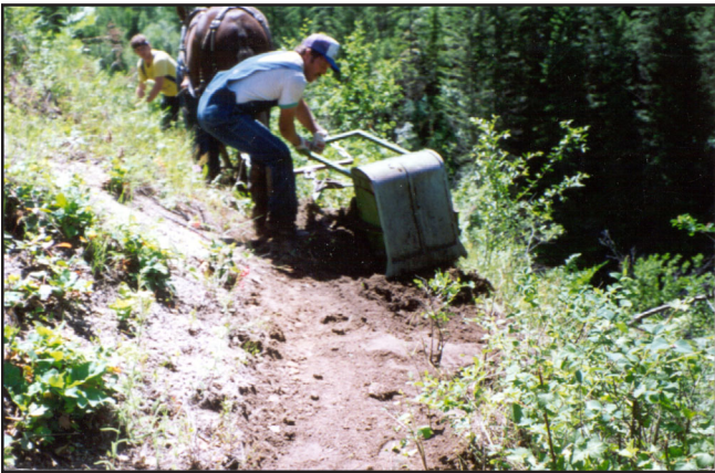
Figure 36—Poor ergonomics of the Trail Ace and Trail Scoop.
