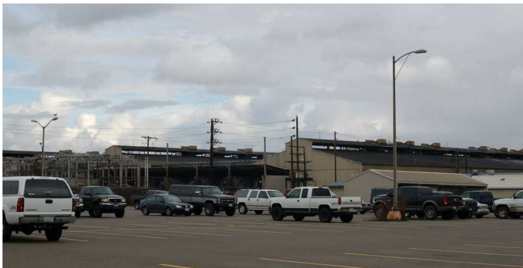
“Potline” buildings at the Alcoa/Intalco aluminum smelter in Ferndale, Washington.
