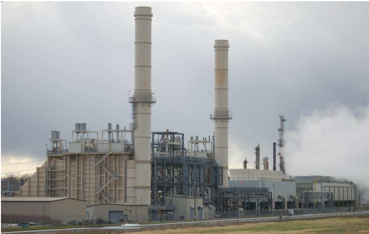
Combined-cycle (gas turbine plus steam turbine) power plant, fueled by natural gas, in Ferndale, Washington.
