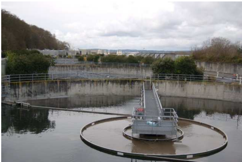
Wastewater clarification at West Point treatment facility in King County (Seattle), Washington.
