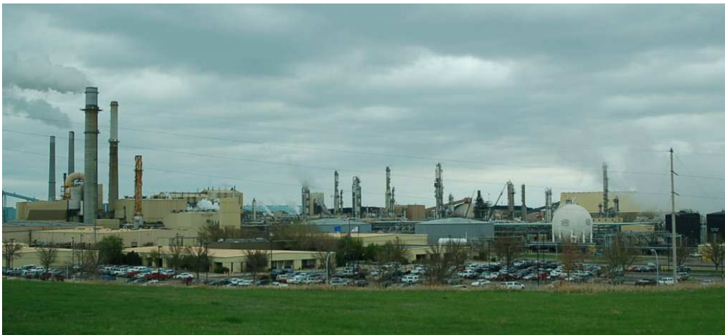
Dakota Gasification plant in Beulah, North Dakota. Produces synthetic natural gas, ammonia, and a variety of other high-value chemical products from coal. A majority of the carbon dioxide produced in this process is captured and piped to oil fields in Canada for enhanced recovery operations, where the CO 2 gas ends up sequestered in underground wells.
