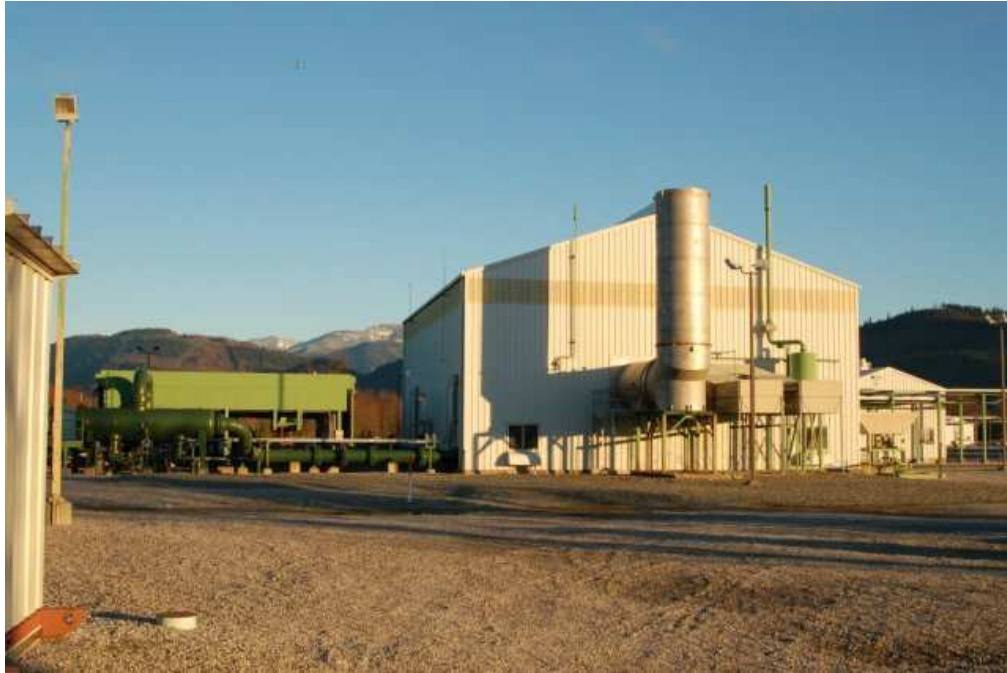
Williams Northwest Pipeline's gas compression facility in Sumas, Washington.
