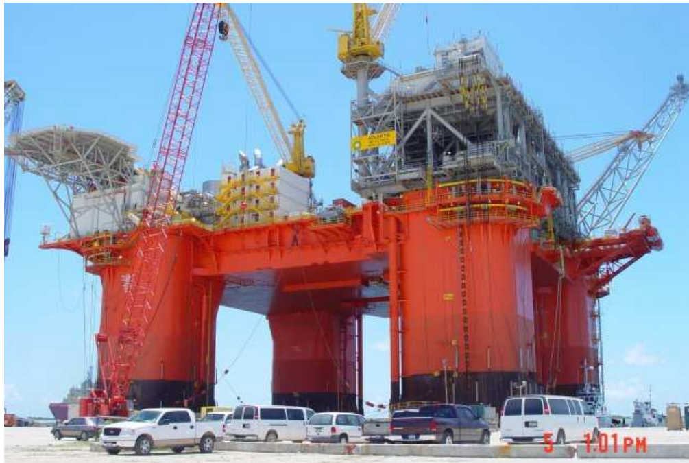
BP Exploration's "Atlantis" offshore rig while under construction.
