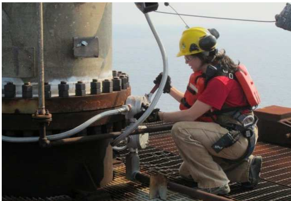
BTC Instrumentation grad Paige repairing flare ignitors on an offshore rig in the Gulf of Mexico.
