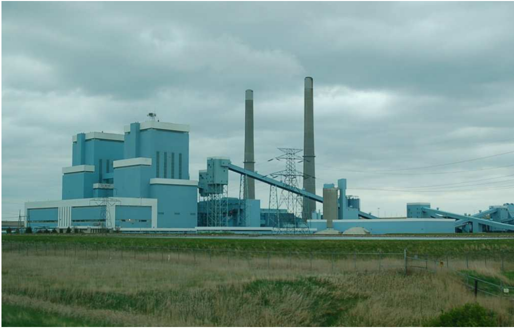
Antelope Valley coal-fired power plant in Beulah, North Dakota.
