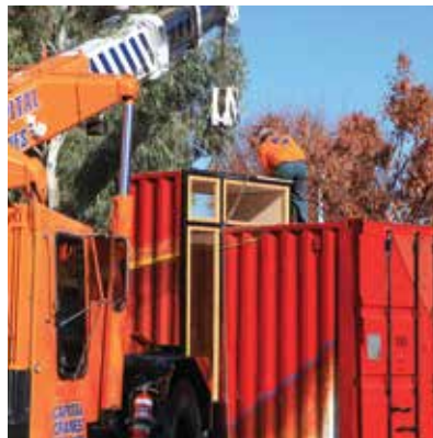
Pop-up shipping container gallery 'Mazz' is craned into location
