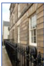
2. Railings outside 79 North Street.
