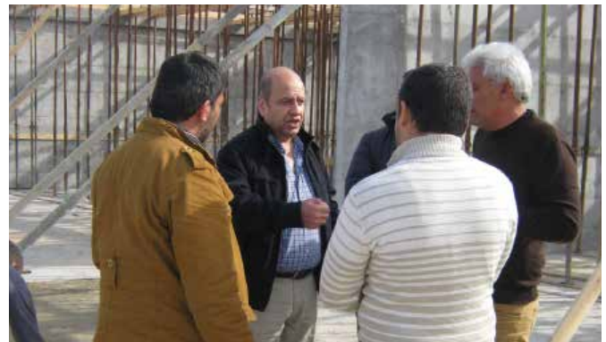
Eng. Munir Manneh speaks with workers at Gaza Bridge Construction Site.
