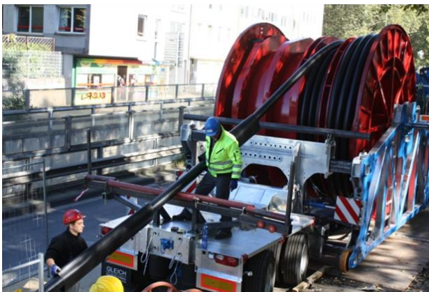
Figure 6 Pulling of first cable length from joint bay
