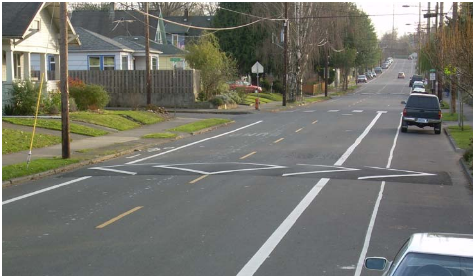
Figure 1: Speed hump on residential street with parking and bicycle lanes in Portland, Oregon
