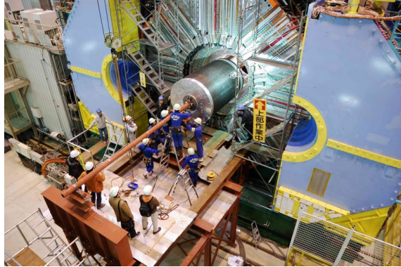
Figure 2: Construction of the Belle Detector
