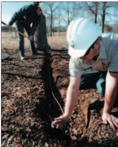
Installing the ground in a trench.
