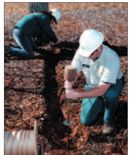
Driving the ground.
