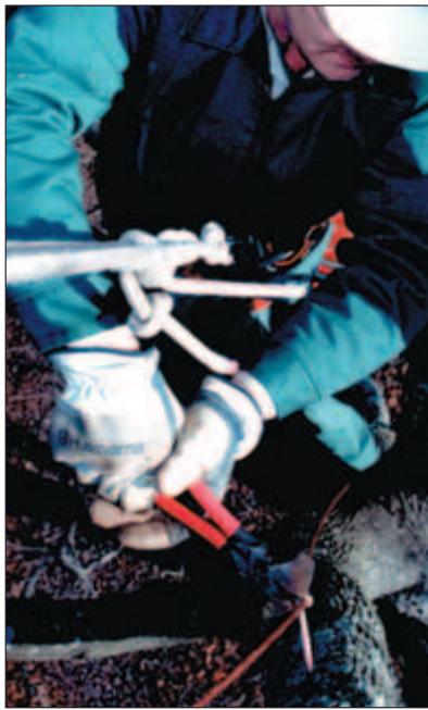
Closing the drive fastener: Drive fasteners are used to secure the conductor to the tree. After it is driven into the xylem, the crimp connector portion of the fastener is closed over the conductor using either a large pair of pliers or as shown in this photograph, fence pliers.
