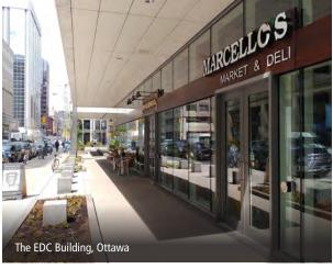
**Figure 3-22:** The cantilevered base building provides a continuous protected area along the building frontage for pedestrians and businesses.
