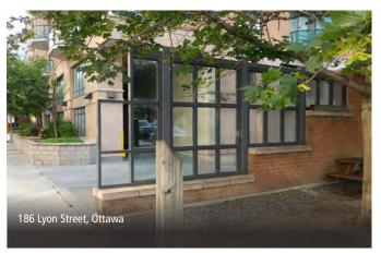
Figure 3-15 A carefully designed feature wall that is integral to the overall architectural expression serving as a screen for the loading and garage entrance.
