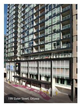
**Figure 2-16:** An example of using architectural articulation to clearly define the base and the middle
