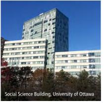
**Figure 2-20:** An example of integrating the mechanical penthouse into the overall architectural design expression.
