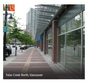
**Figure 3-21:** A continuous canopy is used to protect pedestrians from elements.
