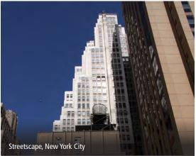
**Figure 3-19** A high-rise building that features significant step backs can open up skyviews and effectively mitigate shadow and wind impacts on the public realm.
