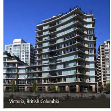
**Figure 2-17:** Horizontal slabs help reduce solar gain in the summer and create a strong rhythm on the facade.
