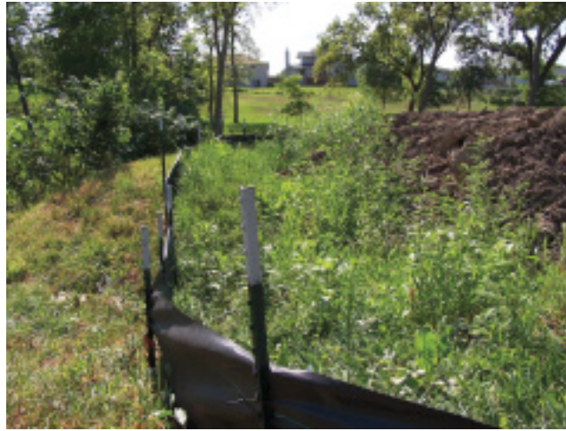
Figure 3.10: Silt fences collect sediment and keep it from reaching water bodies near construction sites. Construction is just starting on this site.
