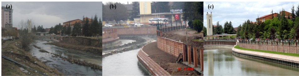
Figure 25. Porsuk Stream in Eskişehir in Turkey Porsuk Çayı (a) before; (b) in application; (c) now (Eskişehir Greater Municipality, 2006)
