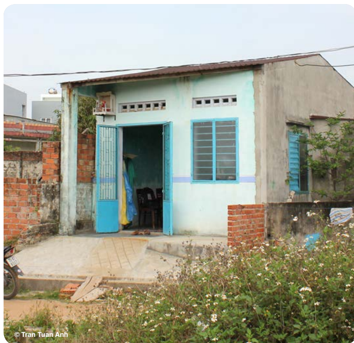
A post-disaster house built after typhoon Xangsane (2006) in Central Vietnam
