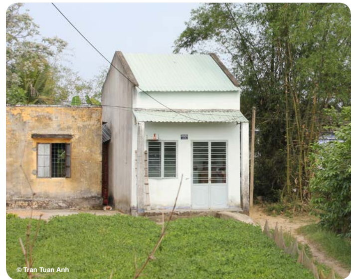
A post-disaster house (white) next to an older model in a peri-urban area of Da Nang City, Central Vietnam
