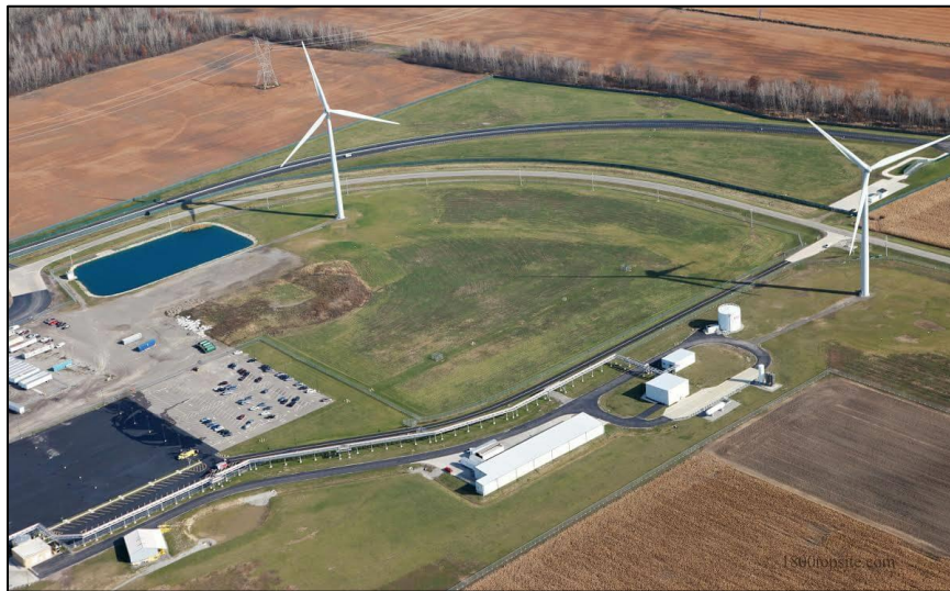
Image 3: The Honda transmission plant in Russells Point, Ohio has two behind-the-meter 1.7-MW GE wind turbines to power its facility. Honda has an interconnect agreement with Logan County Electric Cooperative and a power purchase agreement with Buckeye Power, Inc.
