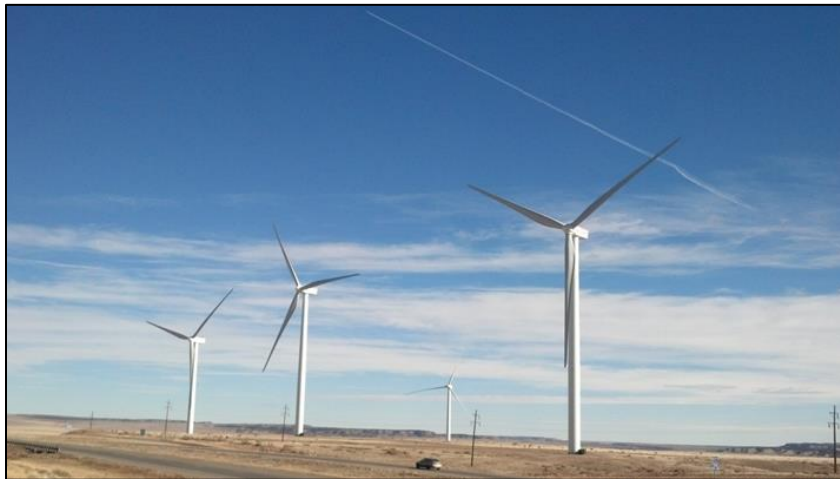
Image 1: San Isabel Electric Association in Colorado purchases energy from the 8-MW Huerfano River Wind Farm. The front-of-meter project includes four 2-MW Sany wind turbines.
