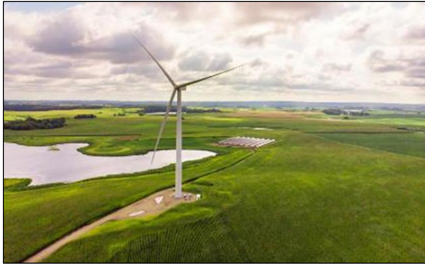
Image 2: The Lake Region Community Hybrid project located in Trondhjem Township, Minnesota includes a 2.3-MW GE wind turbine and 500-kW of solar PV. The energy produced is purchased under a PPA and distributed over local co-op power lines from a single rural substation to Lake Regions Electric Cooperative members. The cooperative is also piloting control technology on 40 large residential electric water heaters to allow them to be charged with off-peak wind power. Real-time data ensures that power from the co-op's wind turbine is serving the program's 80- and 100-gallon water heaters. Photo Credit: Lake Region Electric Cooperative
