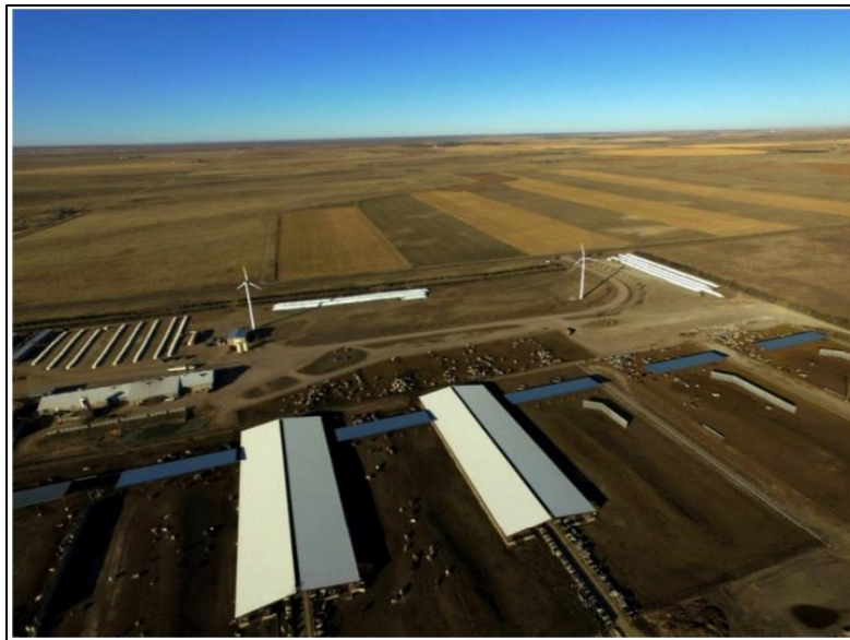
Image 4: The Heritage Dairy Farm owner uses two Northern Power Systems 100-kW wind turbines to provide behind-the-meter energy for the farm's operations in Colorado. The owner also has a 25-kW Eocycle wind turbine at another nearby cattle facility. All three turbines are interconnected to the Y-W Electric Association. Photo credit: Hoss Consulting
