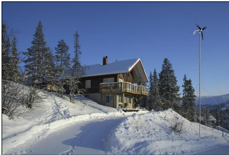
Image 5: Distributed wind can be deployed to power off-grid energy needs. This Primus Wind Power small wind turbine, less than 1 kW in size, powers a remote cabin. Photo credit: Primus Wind Power
