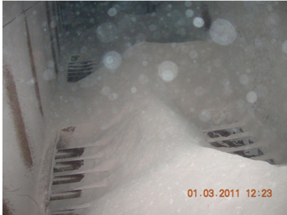
Figure 2.2: Looking into Baghouse
