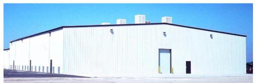
Figure 2: Large scale evaporatively cooled storage facility for cured sweet potatoes. (Photo credit: Robert Kasmire)
