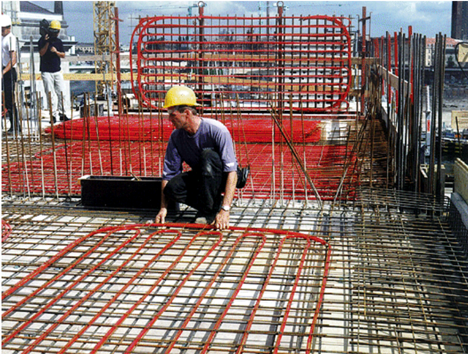
Horizontal loop systems within/beneath slabs
