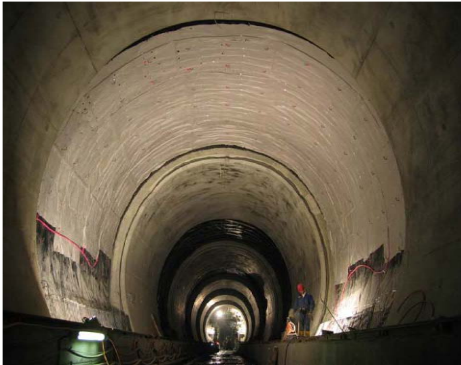
Energy tunnel/anchor systems (Brandl 2006)
