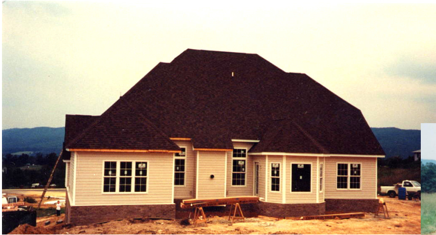
Recently built house in Blacksburg, VA with a trench loop system
